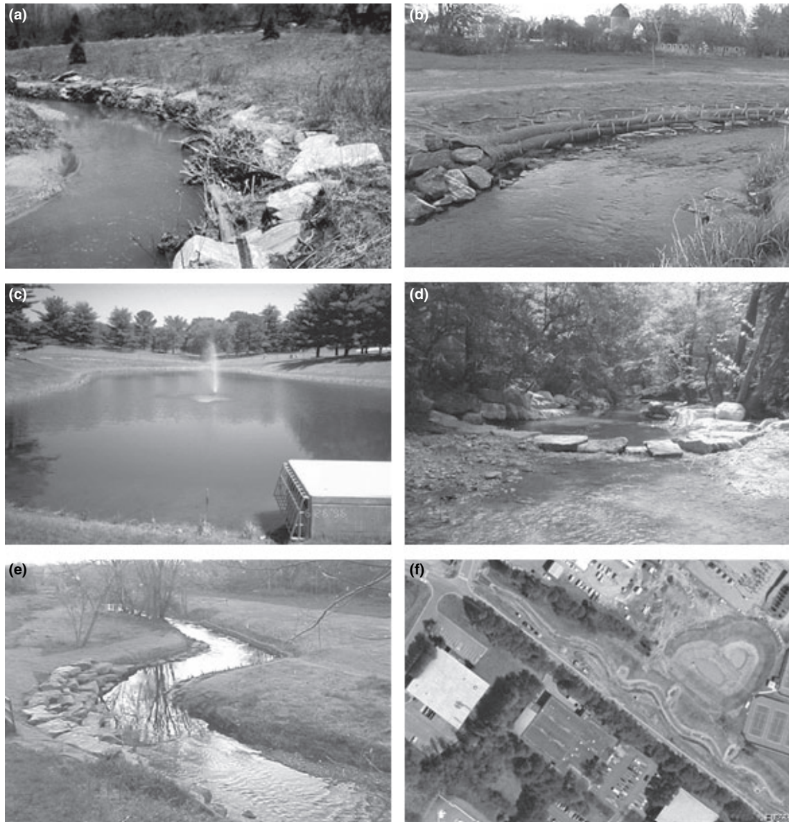
Fig. 6 Examples of common restoration approaches: (a) bank stabilisation of a meander bend with boulders and root wads; (b) bank stabilisation of a meander bend using coir logs; (c) a typical stormwater pond in a new development in a suburban area in MD, U.S.A.; (d) a grade control structure; (e) a channel reconfiguration with reshaped/regraded banks and a meandering channel; (f) a channel reconfiguration and multiple stormwater retention and detention basins along with a large constructed wetland at a severely constrained stream restoration site in Raleigh, NC, U.S.A. (aerial photograph from USGS TerraServer).
